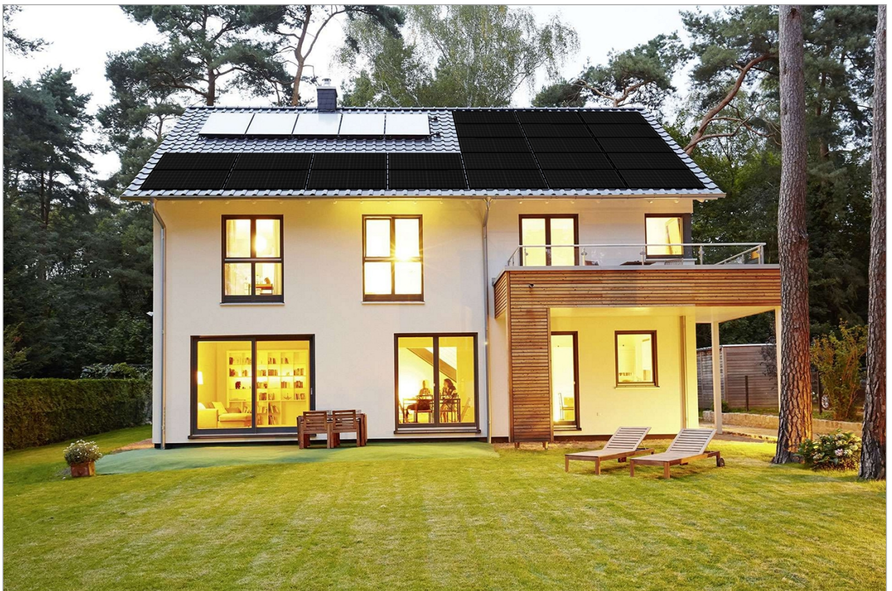
Figure: Photo Preview, 1. Module Area - Modulfläche 1
