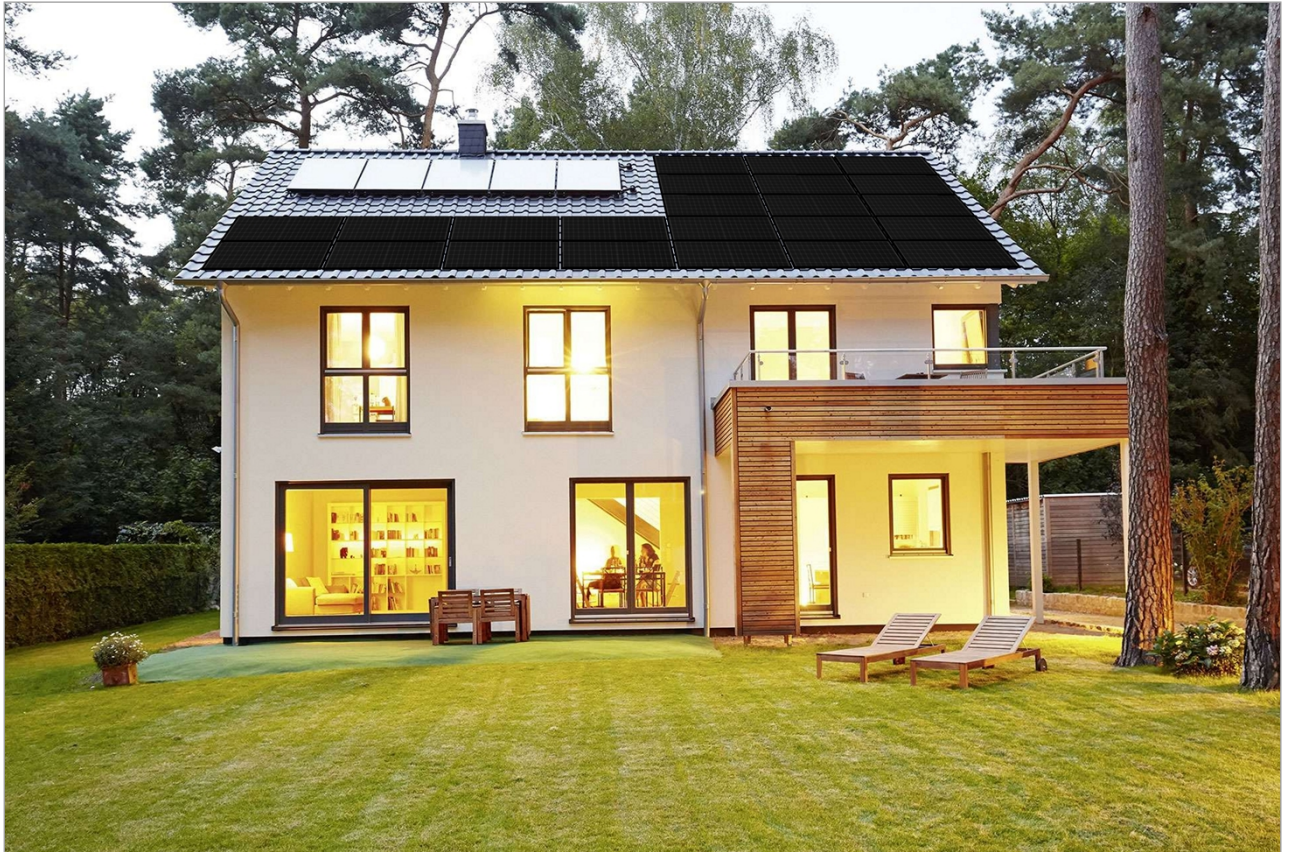
Figure: Photo Preview, 1. Module Area - Modulfläche 1
